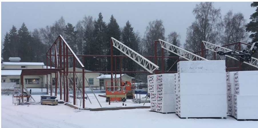
Figur 33. Stomme under montage, objekt 2.
